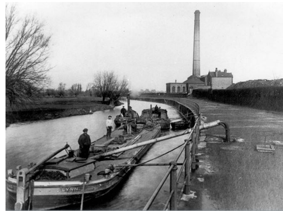
Cambridge bargemen clearing waste from a nearby pumping station
